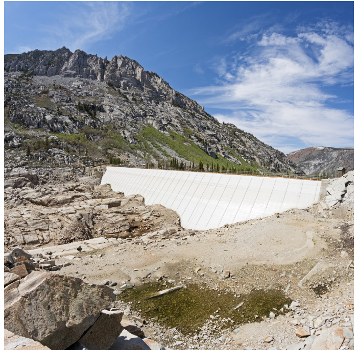
The South Lake Dam in California’s Sierra Nevada shows signs of drought conditions affecting many states in the west.
